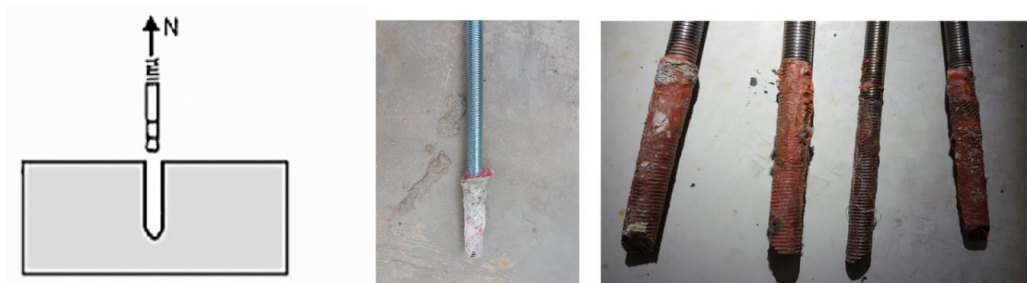
Figure 12. Example of anchor pull-out failure due to improper installation
